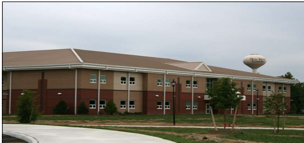
The new high school, a $49.9 million project, was part of the Capital Improvement Program for FY 2008.
